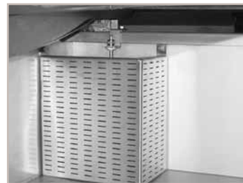
strainer on the pan outlet
